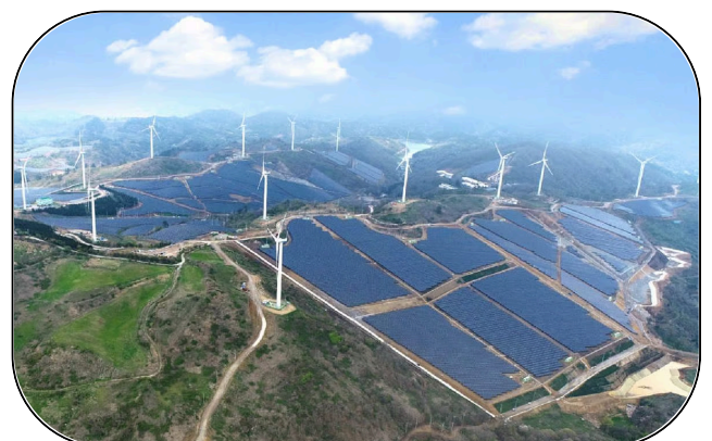
RENEW POWER HYBRID WIND-SOLAR PLANT, KARNATAKA
